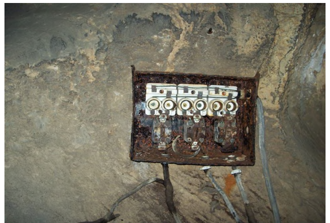
Rusted up switches (John DiCarlo)
