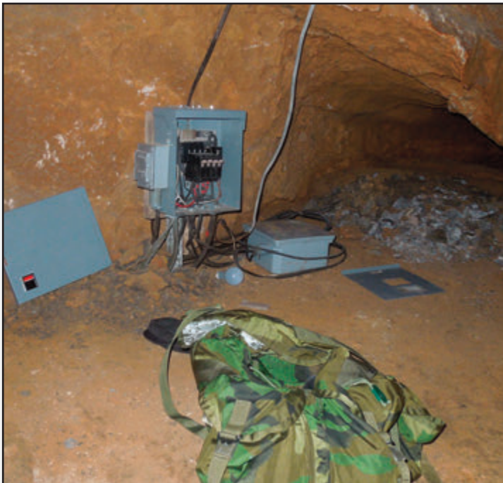
Panel and contactor on the Explorers Loop.
