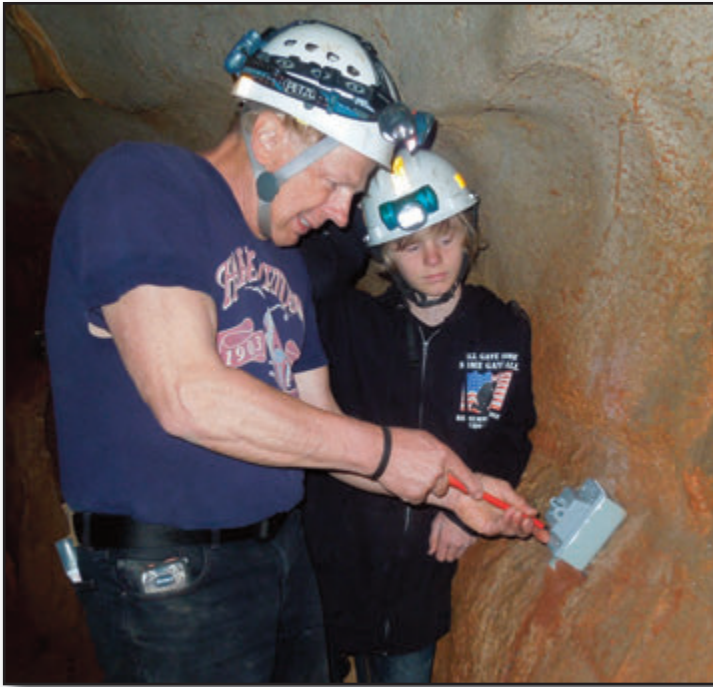
Replacing a three way switch on the commercial trail.
