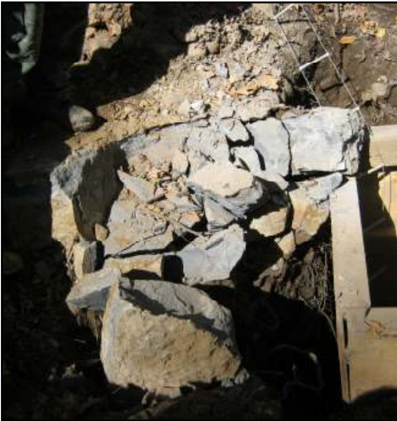
Boulder shattered from 3 straws of chemical persuasion. Ken T
